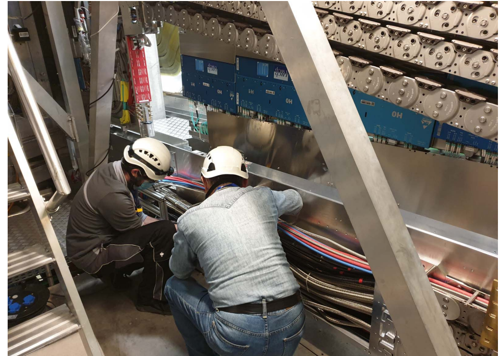
Work on the SciFi tracker installation.
