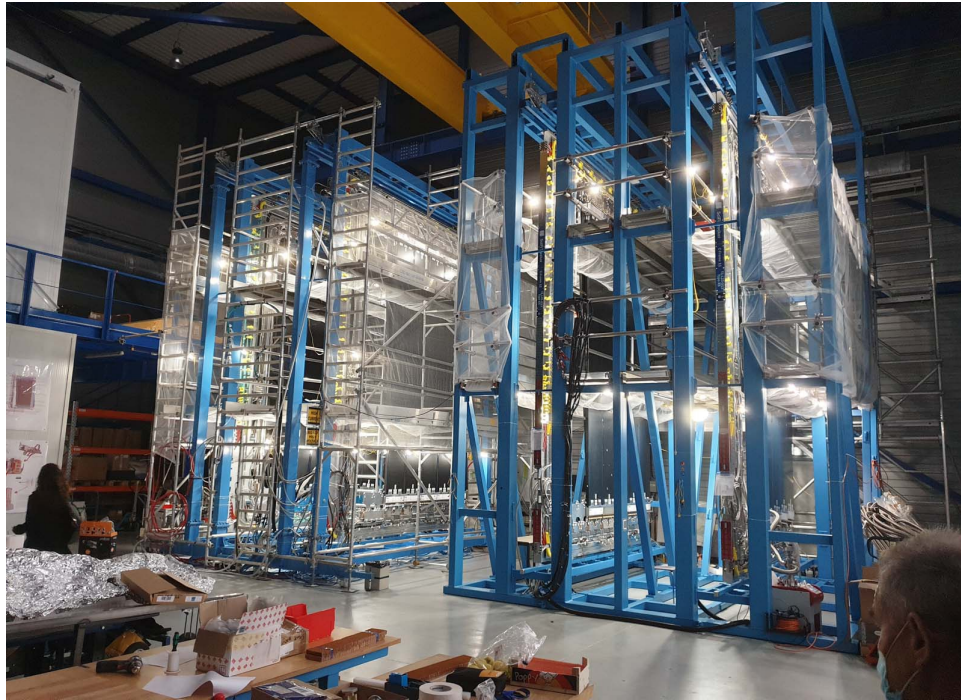
Assembly scaffoldings in the surface building.
