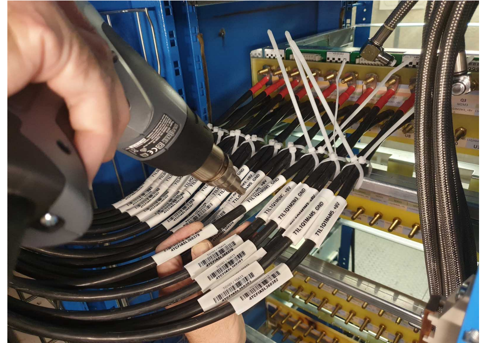
Connecting services and labelling.
