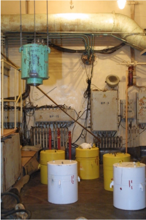
Shielding containers to transport the IBR-30 spent fuel.
