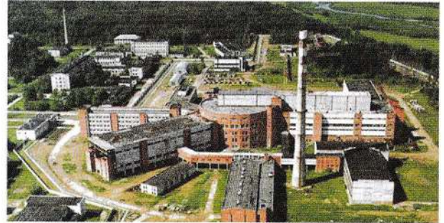
PIK reactor complex buildings
