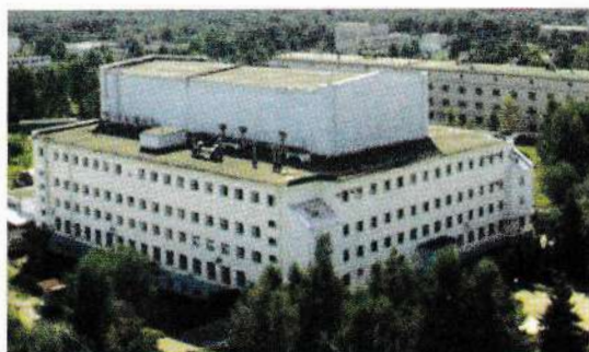
Main building of the SM-3 reactor
