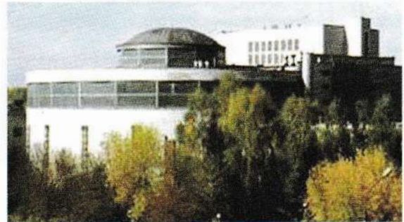
MIR.M1 reactor main building
