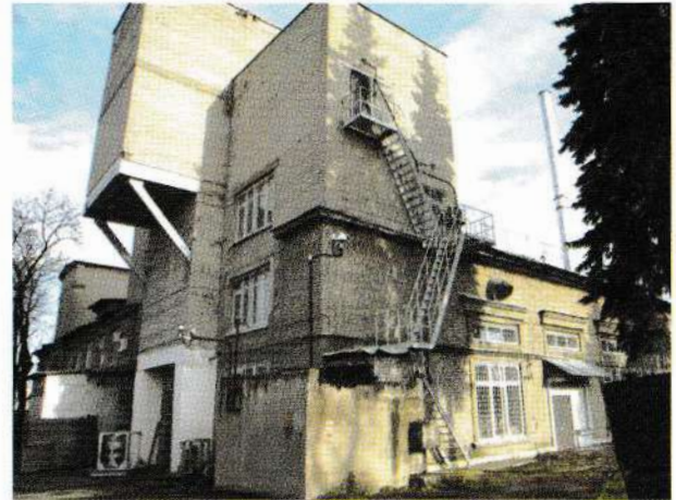
Main building of the IR-8 reactor
