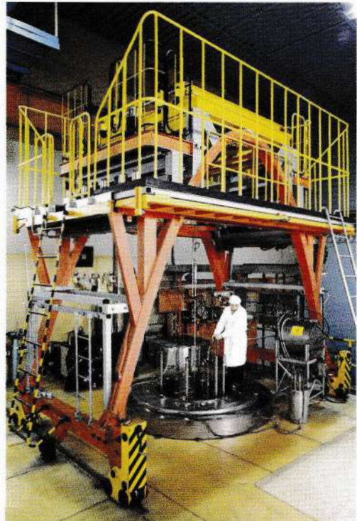
Delta facility compartment
