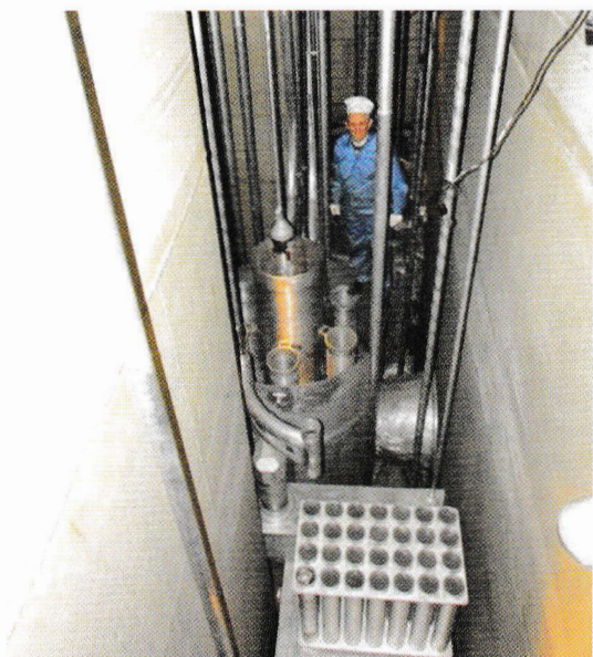
IRV-M2 reactor design inside the pool
