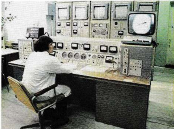
VIR-2M control room
