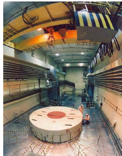
Reactor hall of IBR-2.
