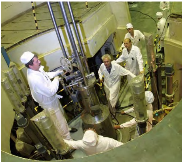
The 22-liter core of IBR-2 with a plutonium dioxide fuel with a critical mass of about 90 kg was placed in the reactor vessel.
