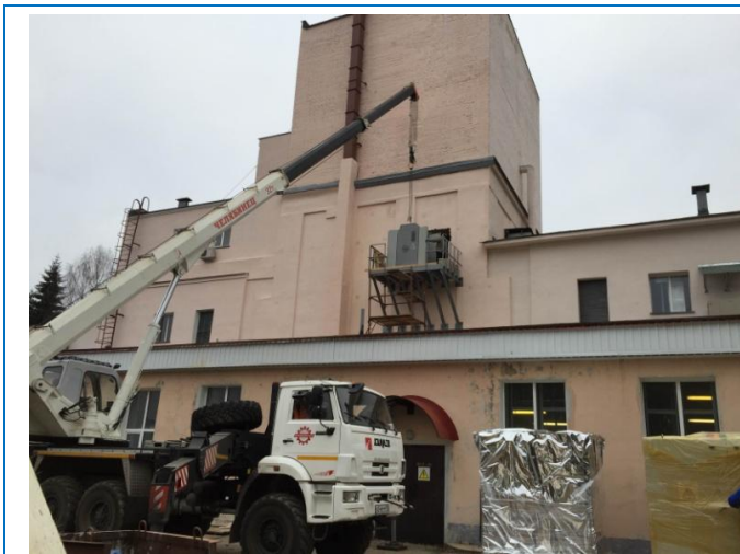
Fig. 27. Lifting of modulators to the accelerator hall through a specially made opening.
