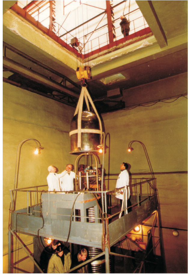
Installation of a high-voltage electrode of the EG-5 accelerator. From left to right: I.A.Chepurchenko, A.P.Kobzev, Zh.G.Ni.
