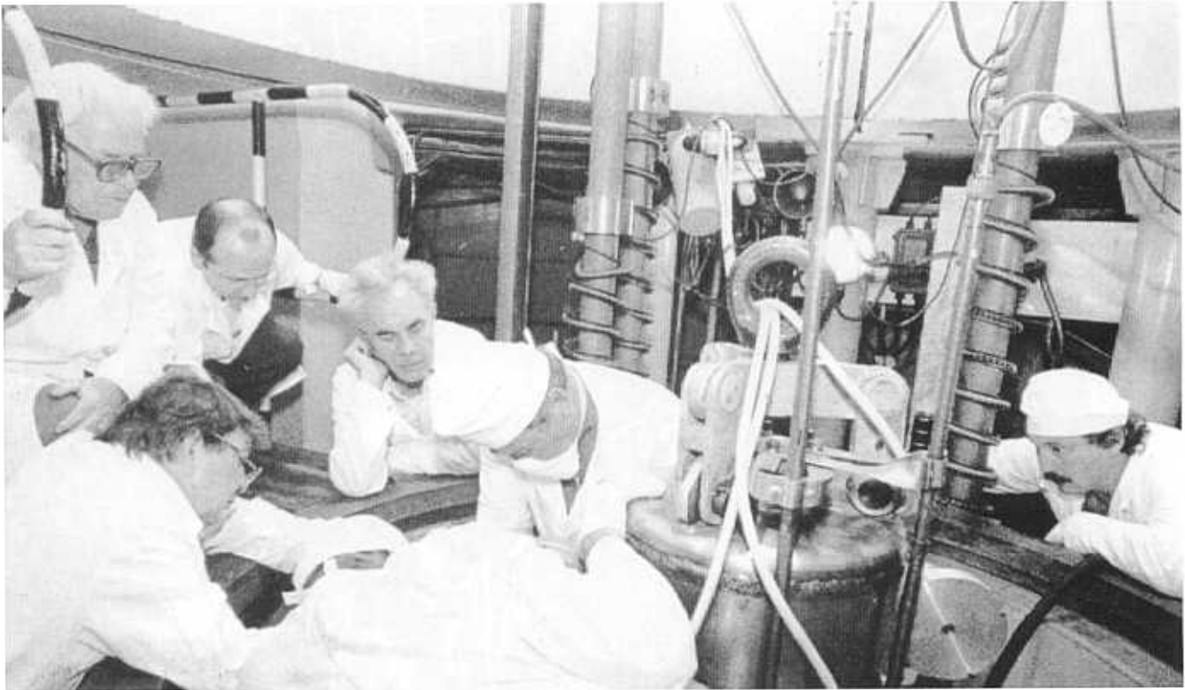
Work to introduce a by-pass into the sodium cooling system of the IBR-2 reactor
