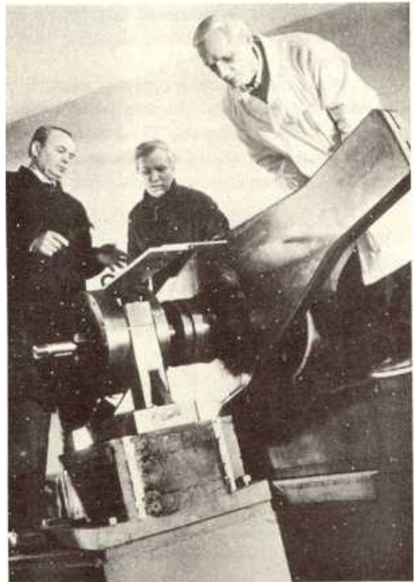
New movable reflector of the IBR-2 reactor
